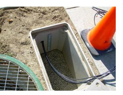
After evaluating the market for a solution, the city turned turned to PPC and adopted its patented Miniflex® pushable fiber cable and ruggedized TuffDuct® microduct, in combination with micro trenching, to bring down the cost and time of last-mile FTTP and FTTH deployments.
